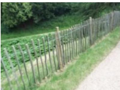
These tend to be used as barriers rather than safety fences as they would be easily climbed and usually have horizontal rails with wide spacing. Strained wires can be
