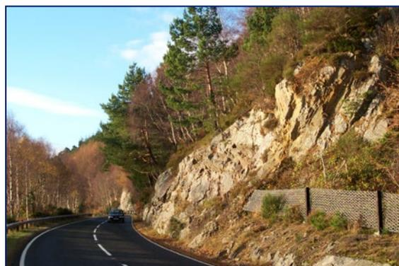
Fig.2 Steel protective fences erected to protect against rock falls and other debris.
