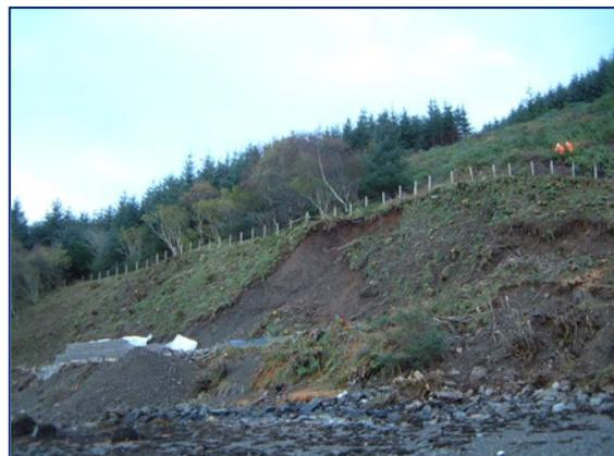
Fig.1 Major landslide on A82 – the road surface is under the rock and earth!
