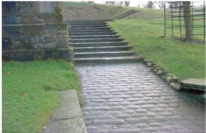
All sealed surface paths including paving, concrete and asphaltic/bitumous surfaces mentioned below require either a camber or cross-fall for drainage purposes. These should not exceed 2.5 per cent (1 in 40) and should not be less than 1 percent.
