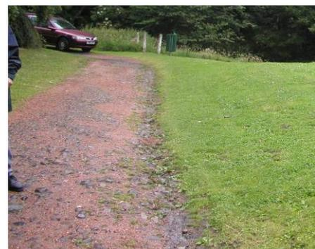
**Grass** – Grass can be slippery when wet; but for paths with little or no gradient, and where light levels are sufficient, and trampling pressure is fairly low, grass makes an attractive path surface, which should be durable on free draining soil.
