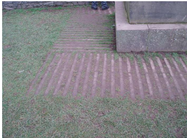
Castellated or studded systems can be difficult for pedestrians as the soil fill within the units settles or is washed from the surface, leaving a protruding 'stud' which presents a significant trip hazard.
