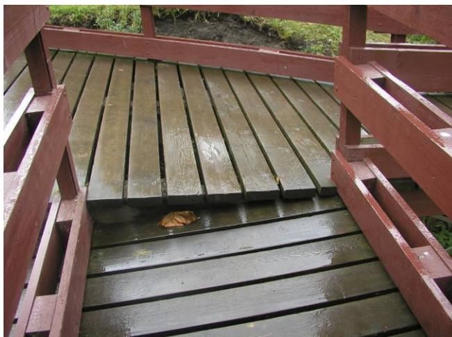
**Timber Decking** – On boardwalks with timber decking, boards should be laid at right angles to the direction of pedestrian flow. For boardwalks used by disabled people there should be a maximum gap between boards of 12mm. A larger gap of up to 25 or 30mm can be used on those installed in more remote and inaccessible locations.
