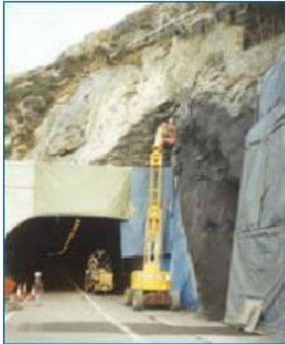
**Spraying reinforced concrete, A55 North Wales**
